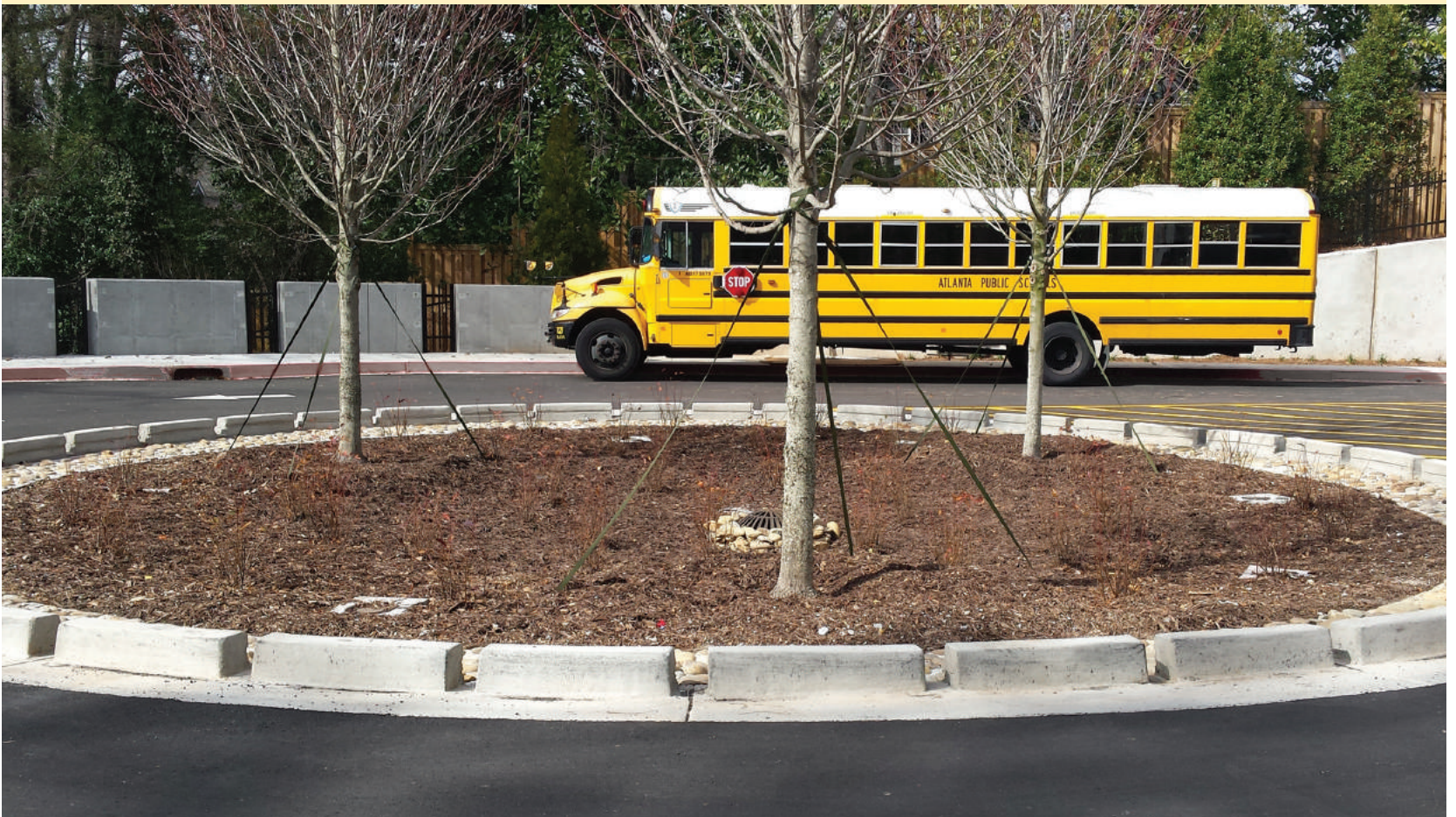
Bioretention cul-de-sac at E. Rivers Elementary School.
